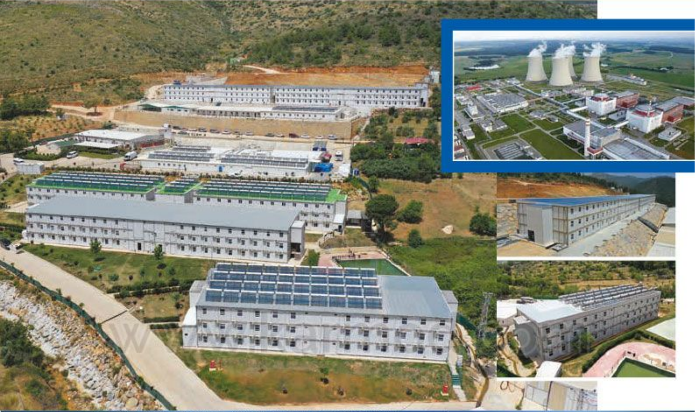
Akkuyu Nükleer Santrali, Mersin • Akkuyu Nuclear Power Plant, Mersin
