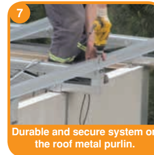
Screw connection system that gives durability to our structures
